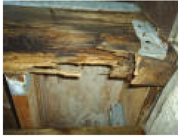
Termite Damage
