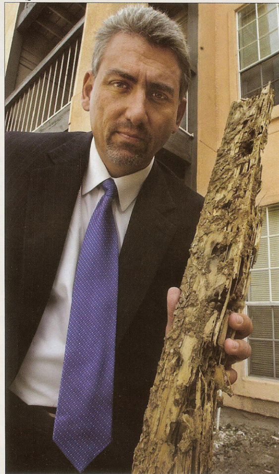
GNAWED: Attorney Pete Cardillo with evidence of termite damage.
